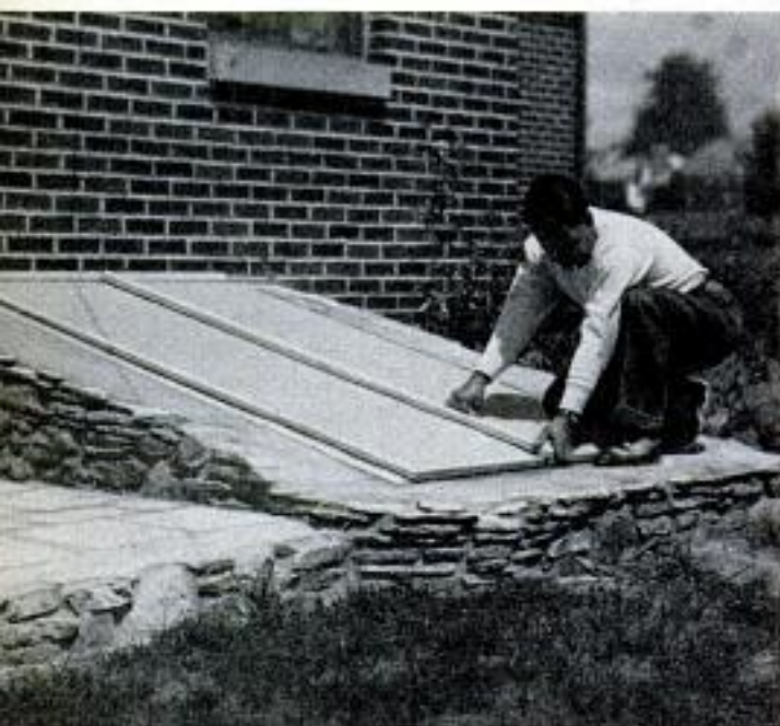
Stone wall around basement entrance blends it with stone-edged patio. Doors are painted to match stone
